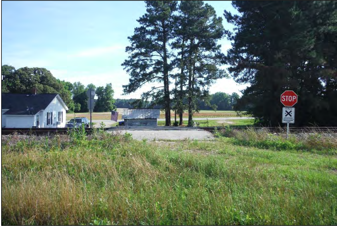
Figure 7. WL2115, dwelling, rear addition, view to the north.
