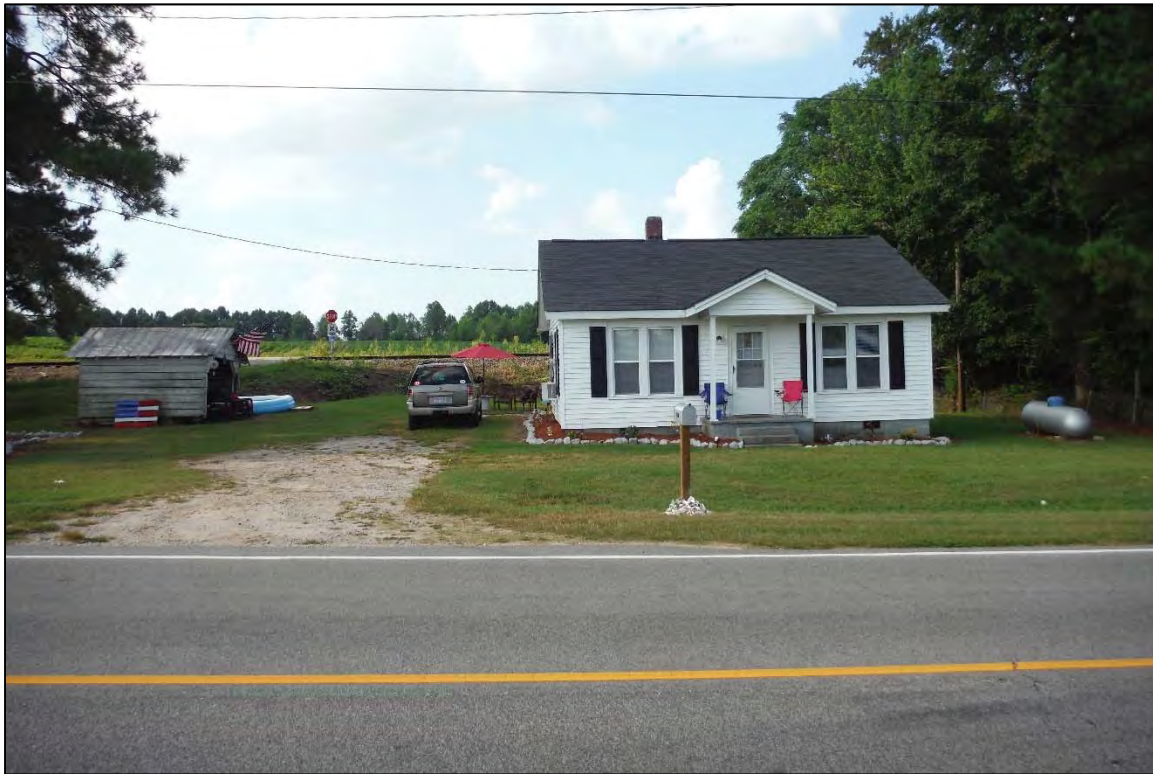
Figure 5. WL2115, dwelling, view to the southwest.
